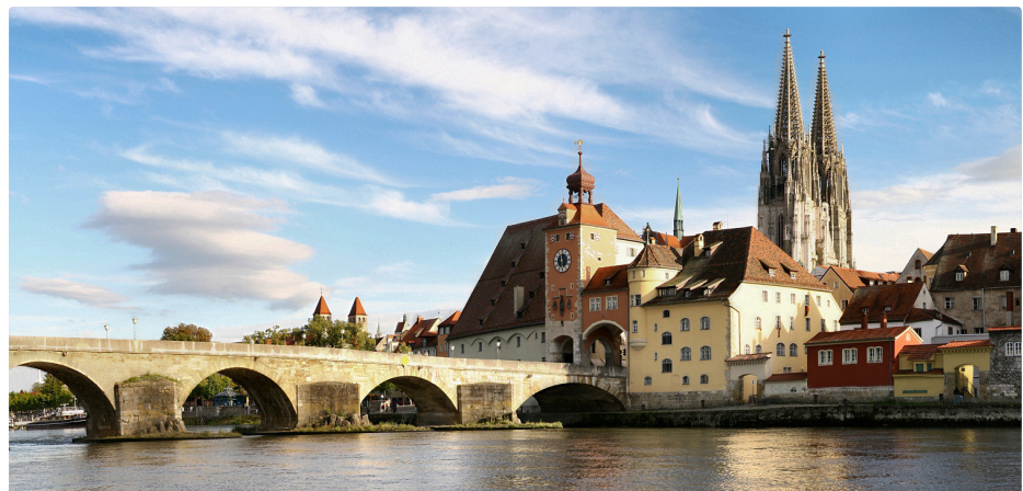
BELOW Typical view at Regensburg.
