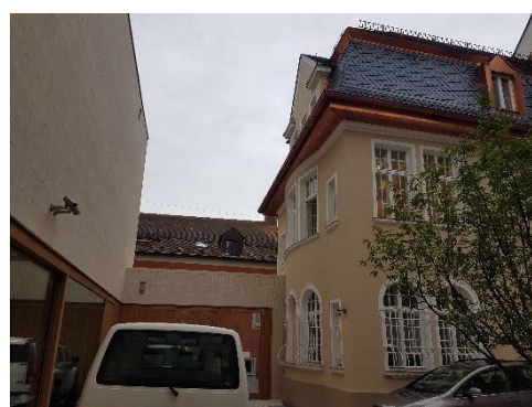
Fig. 4: Workshop location - 1st Floor in the right building.
