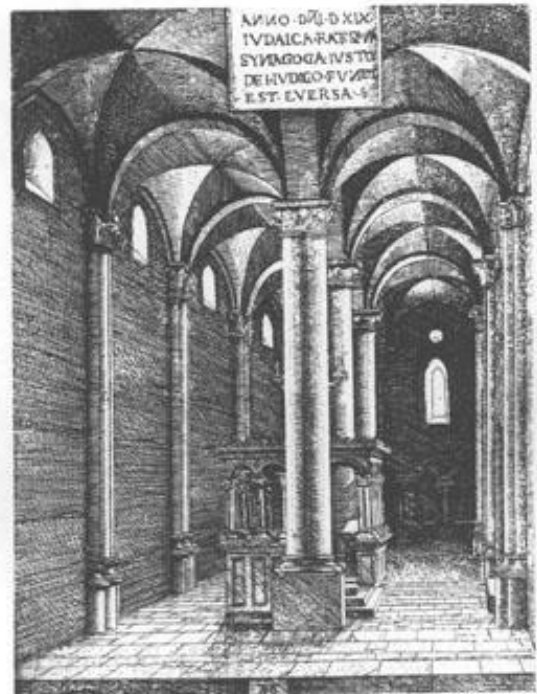
Fig. 13: Etching by Albrecht Altdorfer Regensburg synagogue immediately before its destruction 1519
