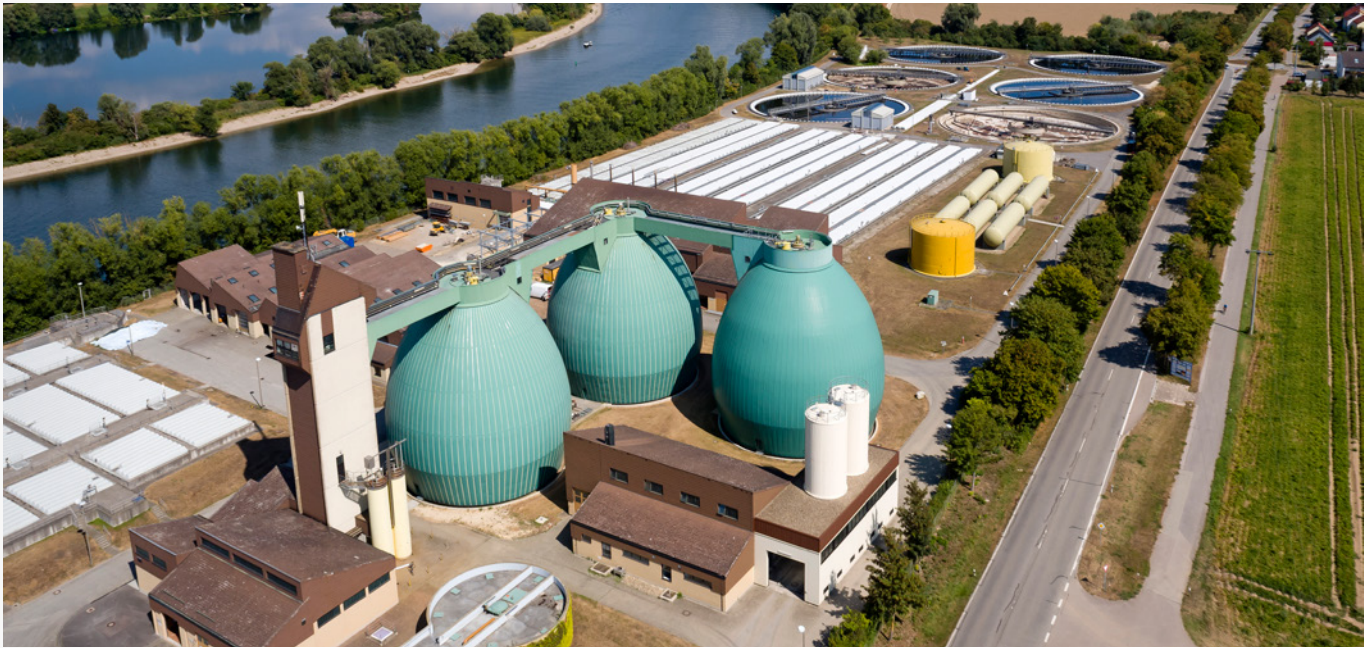
The Regensburg wastewater treatment plant.
