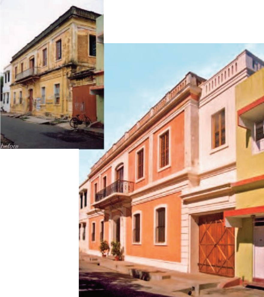
Figure 5 Hotel De l' Orient, before and after restoration (P. INTACH 2008, 15)
