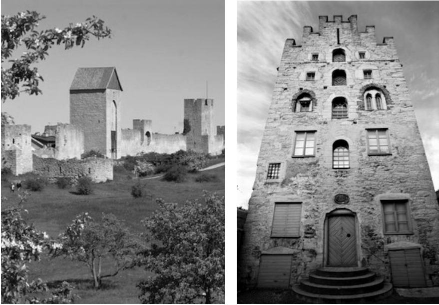
Figure 2: Gamla Apoteket (Old Pharmacy), a medieval warehouse building with a distinctive stepped gable at Strandgatan, built in local limestone in the 13th century. It was used as a pharmacy in the 19th century (Photo: Sara Appelgren, ©Region Gotland and Gotlands Museum).
