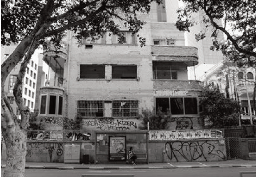
Figure 2: Sample of a dilapidated Bauhaus in zone A (own source)
