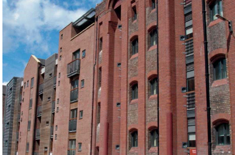
Converted warehouses and sensitive new buildings in Argyle Street, Liverpool
