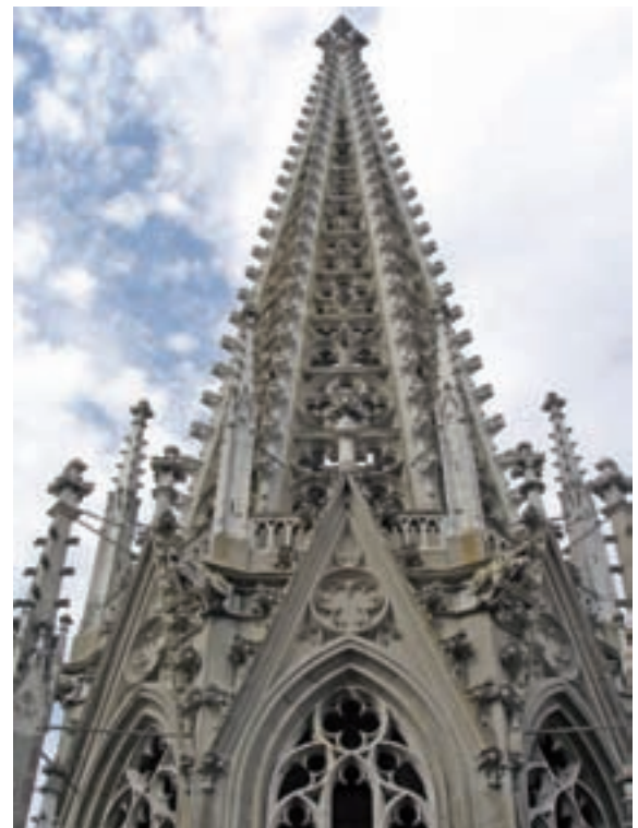
Picture 5: View to the north helm roof of the steeple
