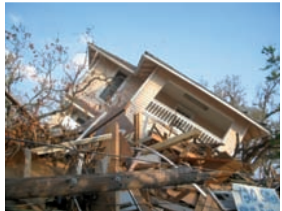
House in Biloxi, USA; damaged by Hurricane Katrina
