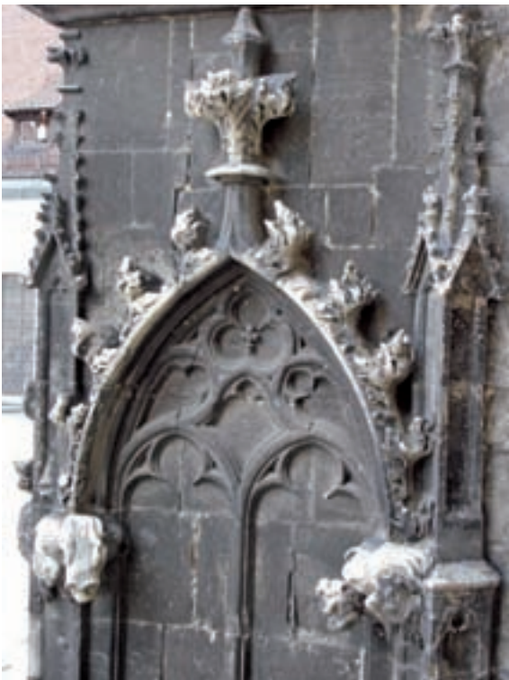
Picture 2: Uncleaned stone surfaces with crust formation
