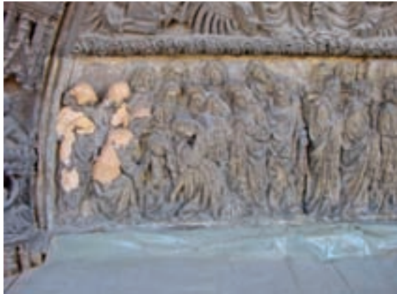
Picture 8: Cleaning the reliefs by means of the ion-exchanger method
