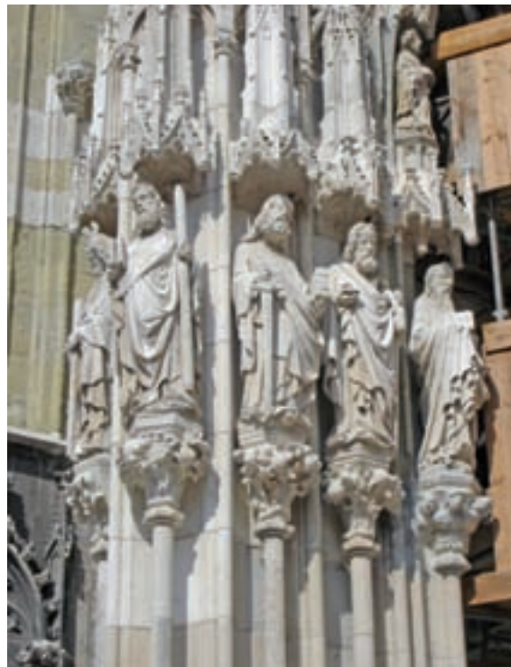
Picture 7: Pillar after cleaning and renovation
