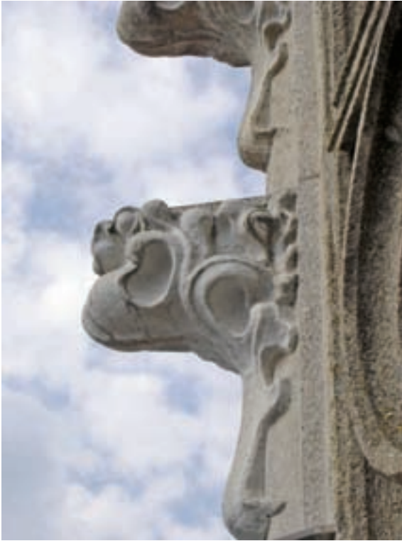
Picture 6: Insertion of a new crocket of cast concrete
