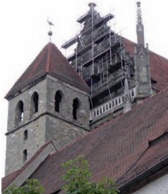
Picture 3: Transept gable with safety scaffold
